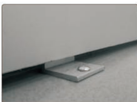
5.1 Fix the anti-sway device (framed glass door)
