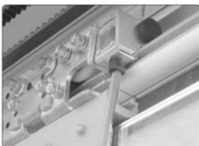
Use wrench to tight the positioning block
