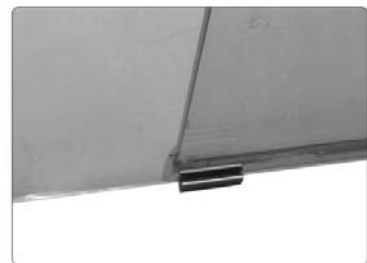
5.6 Fix the anti-sway device on the ground
