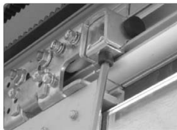
5.5 Use wrench to tight the positioning block
